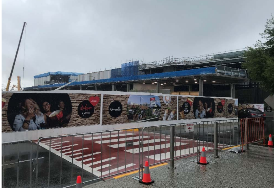
Construction works on Kawana Shoppingworld
